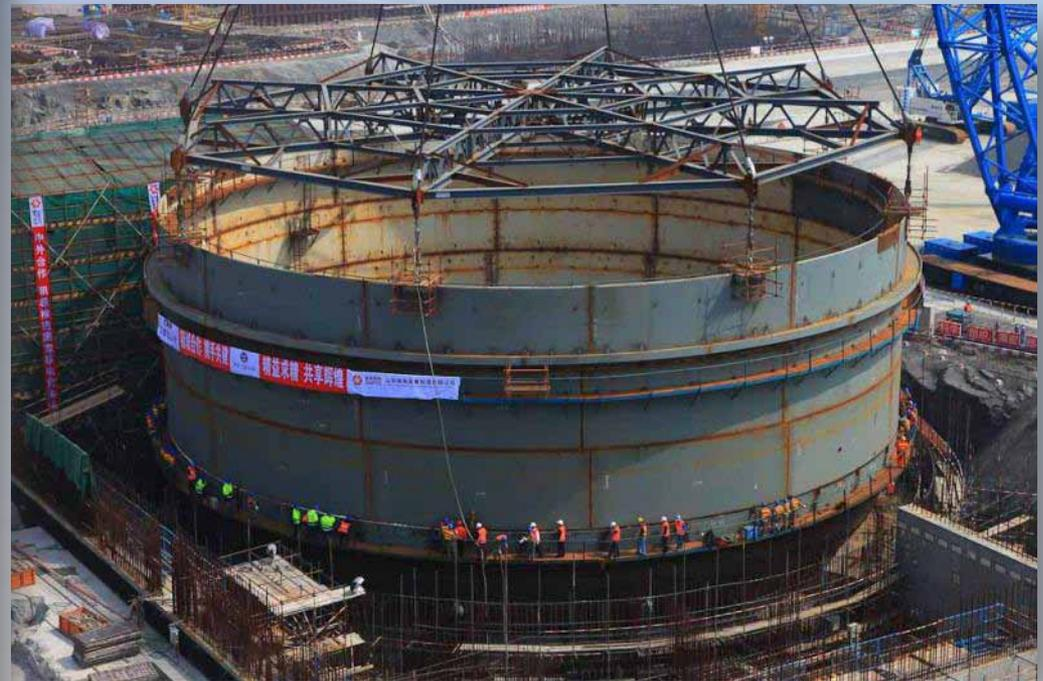
CV 1<sup>st</sup> Ring set into place on CV Bottom Head
