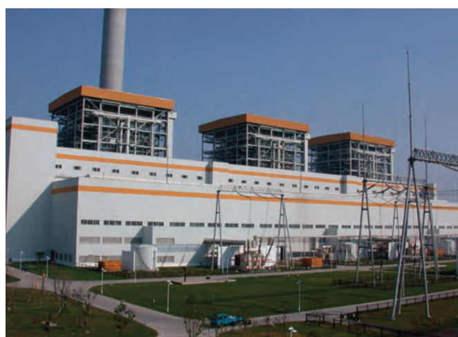
Figure 6 Changshu supercritical pulverised coal-fired power station in Jiangsu Province. The plant uses three 600 MWe once-through SC wall-fired boilers supplied by Doosan (courtesy Doosan Babcock)
