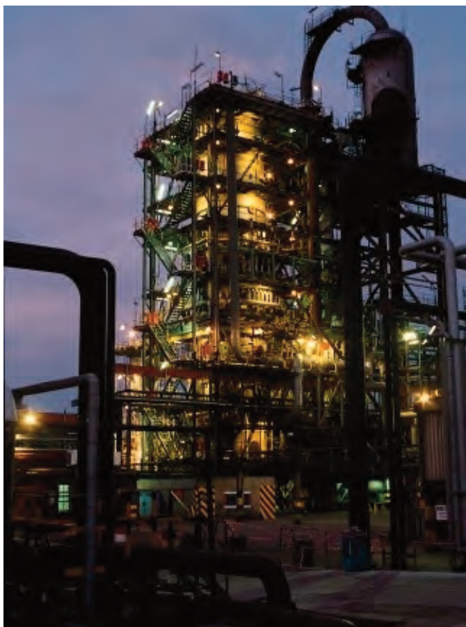
Figure 22 Slurry reactor forming part of Sasol's extensive Secunda CTL plant, reportedly the world's single largest point source of CO 2 (courtesy World Petroleum Congress)
