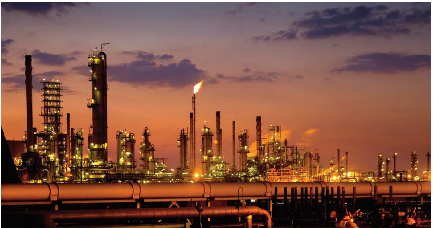
Figure 13 Part of Sasol's Secunda CTL plant (courtesy World Petroleum Congress)
