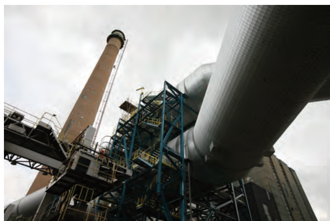
Figure 11 Part of the new FGD facility being added to International Power's Rugeley B coal-fired power plant in the UK (courtesy Russell Mills Photography)
