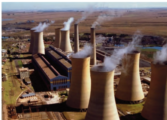
Figure 10 The Komati coal-fired power plant in South Africa. Mothballed in 1990, it is currently being upgraded, refurbished and recommissioned (courtesy Eskom)
