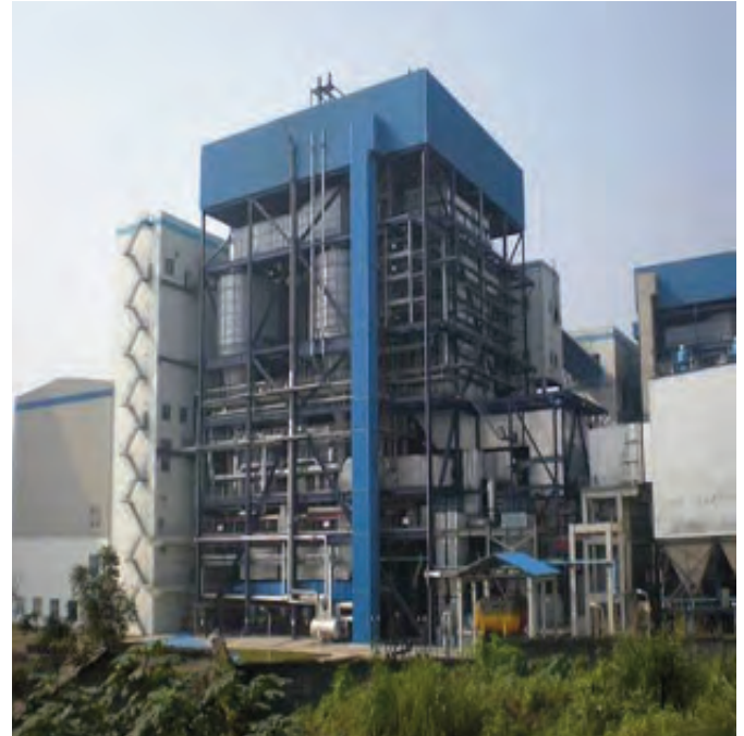
Figure 5 330 MWe CFBC boiler in operation in January 2009 at Fenyi Power Plant
