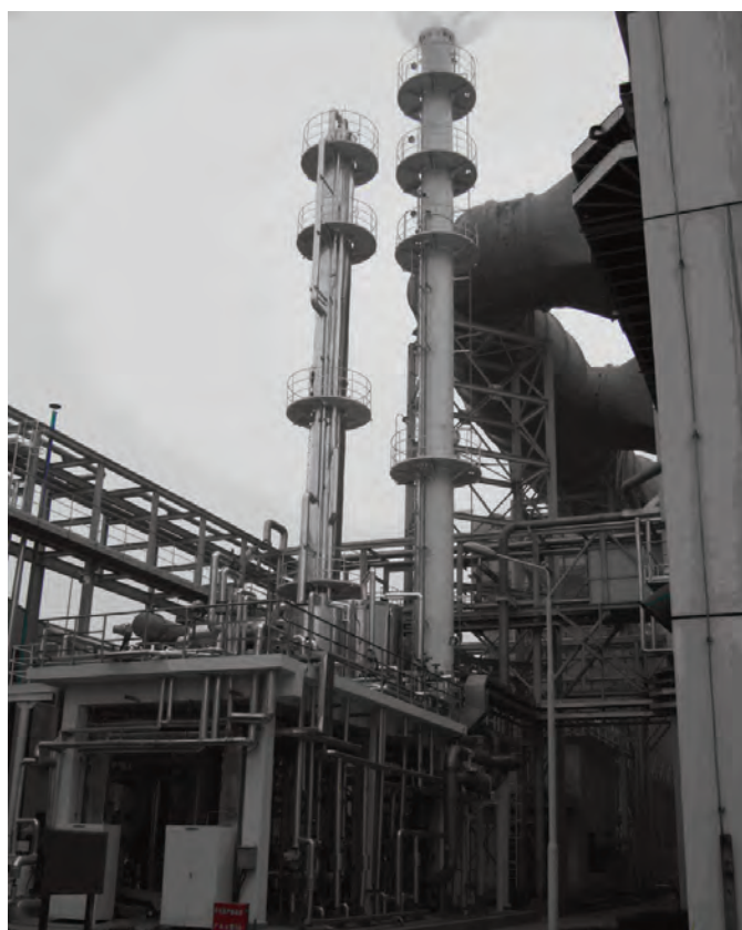
Figure 8 Main structure showing stripper (left) and absorber (right) of the Huaneng post-combustion CO 2 capture pilot unit
