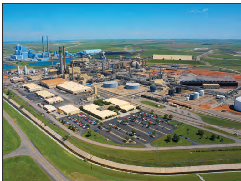
Figure 10 A major lignite consumer is the Great Plains synfuels plant near Beulah in North Dakota. Since 1984, this has been using Lurgi gasifiers to produce SNG and other products. Since 2000, CO 2 has been captured and piped to Canada for enhanced oil recovery applications (photo courtesy of Basin Electric Power Cooperative)
