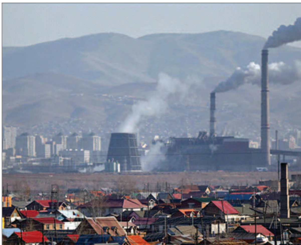
Figure 5 View of one of the elderly coal fired CHP plants in Ulaanbaatar together with various dwellings established by former nomads on the edge of the city (Prophecy Coal, 2012a)
