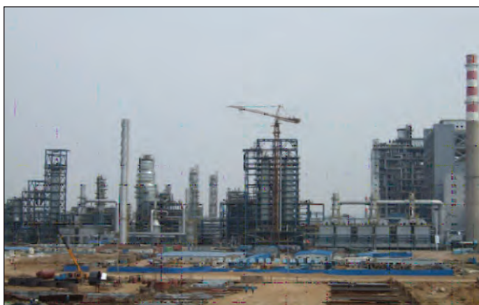
Figure 9 View of the Shenhua DCL production line with construction close to completion (Minchener, 2008)
