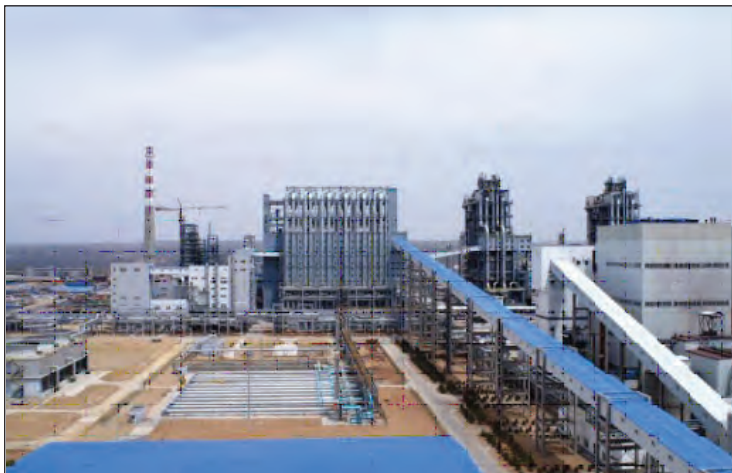
Figure 11 View of the Shenhua Baotou coal to chemicals plant (Baotou News, 2009)
