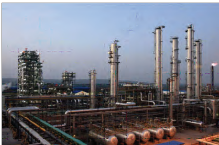
Figure 8 View of the Shanxi Lu'an coal-to-liquids demonstration plant (Synfuels China, 2010b)
