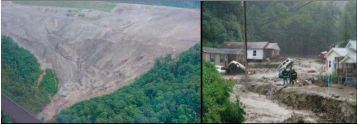
**Figure 19 Lyburn flood (left) erosion and sloughing on the outslope of the durable rock fill following a storm event; (right) property damage downhill of the fill (Michael and others, 2009)**
