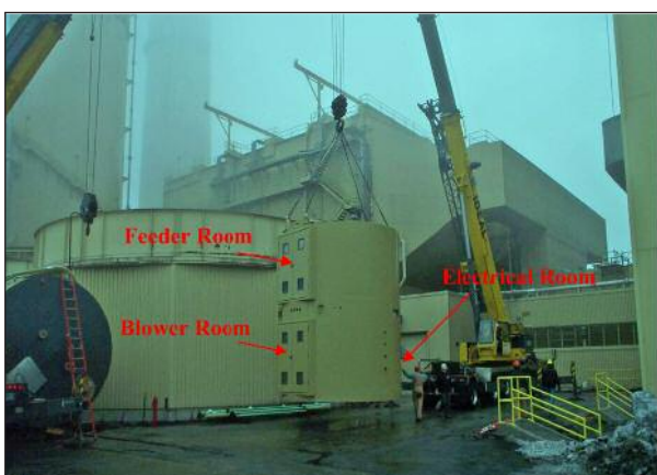
Figure 14 Installation of process equipment model at Edgewater Unit 5 (Starns and others, 2011)
