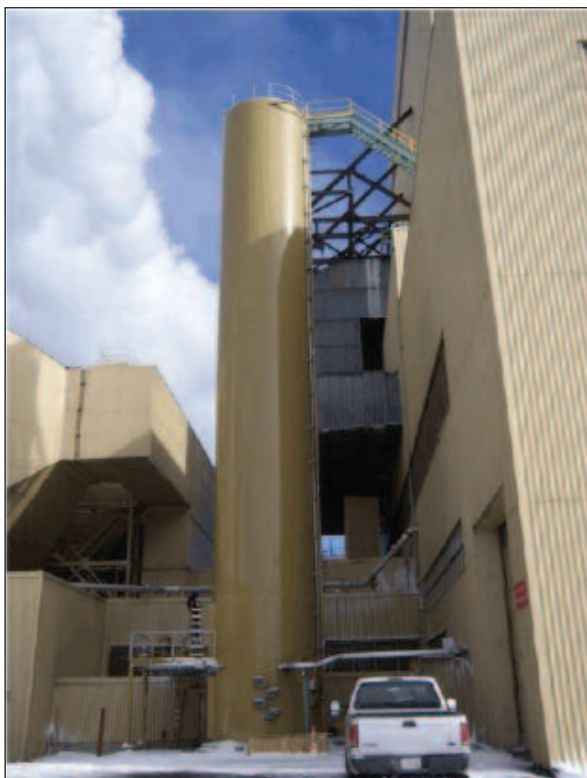
Figure 13 Edgewater Unit 5 ACI system silo (Starns and others, 2011)
