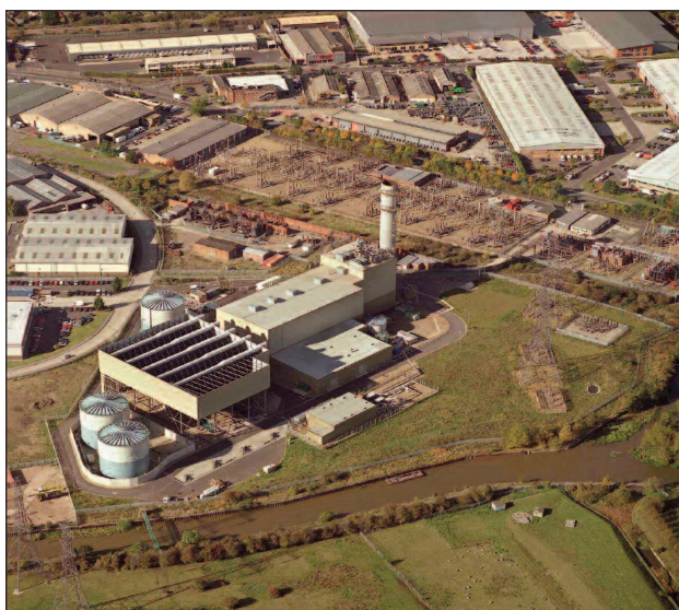
Figure 6 Gas-fired combined cycle plants are often used to respond quickly to changes in electricity demand (photograph courtesy of E.ON UK)
