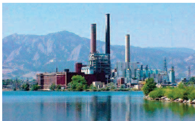
Figure 16 The Cameo Generating Station, Colorado, USA. This coal-solar hybrid uses parabolic trough solar collectors to collect sunlight (photograph courtesy of Xcel Energy)
