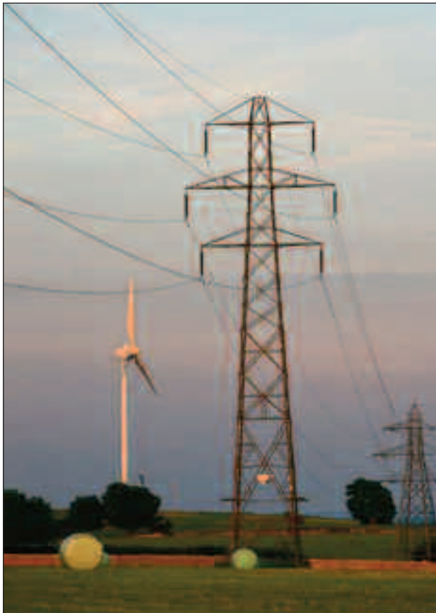
Figure 4 Wind turbine, UK. A 500 kW gearless Enercon turbine. Annual output clearly depends on prevailing weather conditions (photograph courtesy of Russell Mills Photography)
