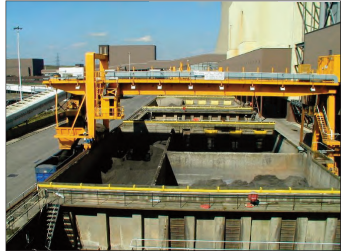
Figure 3 FBA collection pits at a coal-fired power station (photograph courtesy of UKQAA, 2009)
