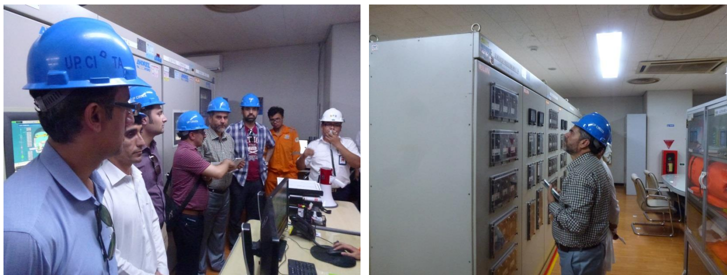
(Left) The delegation learns about the Java-Bali interconnection system. (Right) DABS Director of the Takhar Region, Mr. Mohammad Momand inspects the control room at the Cirata Hydroelectric Power Project.
