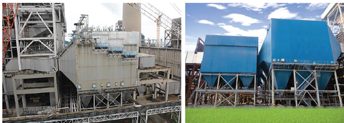
Figure 15 Feida EFF system at Huaneng Taichang, left, and Anpeila, right, power plants ( www.feida.biz )
