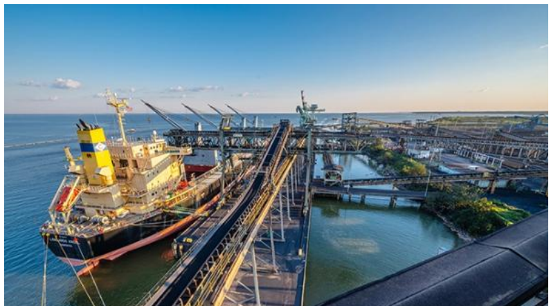
Image 1. McDuffie Coal Terminal at the Port of Mobile, Alabama. Source: Alabama Port Authority, Coal, Port of Mobile Facilities
