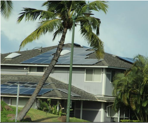
Residential solar panels on a rooftop in Oahu.
