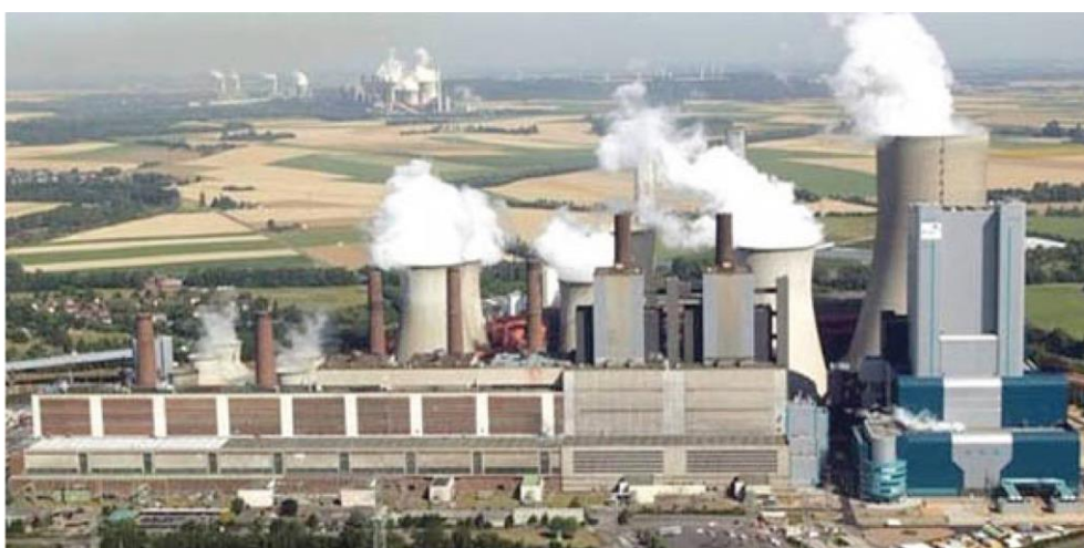
Figure 2 RWE's 3.68 GW lignite-fired Niederaussem power plant in Germany (photograph courtesy of RWE)
