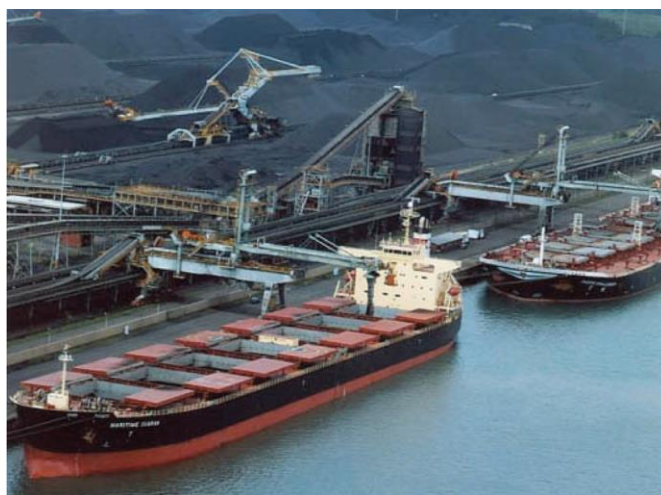
Figure 10 The Richards Bay coal export terminal (photograph courtesy of Richards Bay Coal Terminal Proprietary Ltd)
