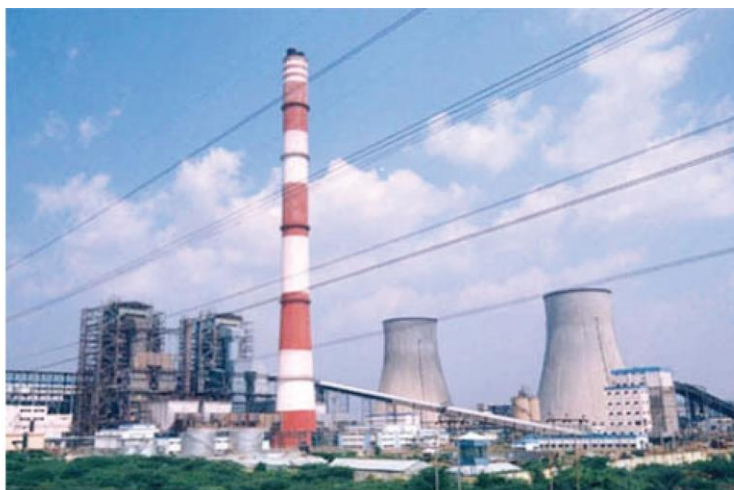
Figure 1 The 250 MW CFBC power plant of Neyveli Lignite Corporation (NLC) in Tamil Nadu (photograph courtesy of NLC)
