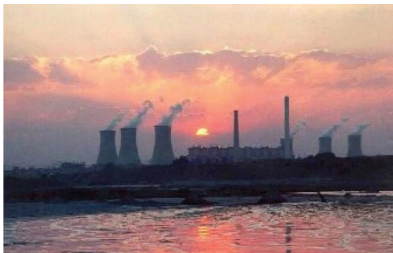
Figure 11 Eskom's 3.6 GW base load coal-fired Matla power plant, South Africa (photograph courtesy of Eskom)
