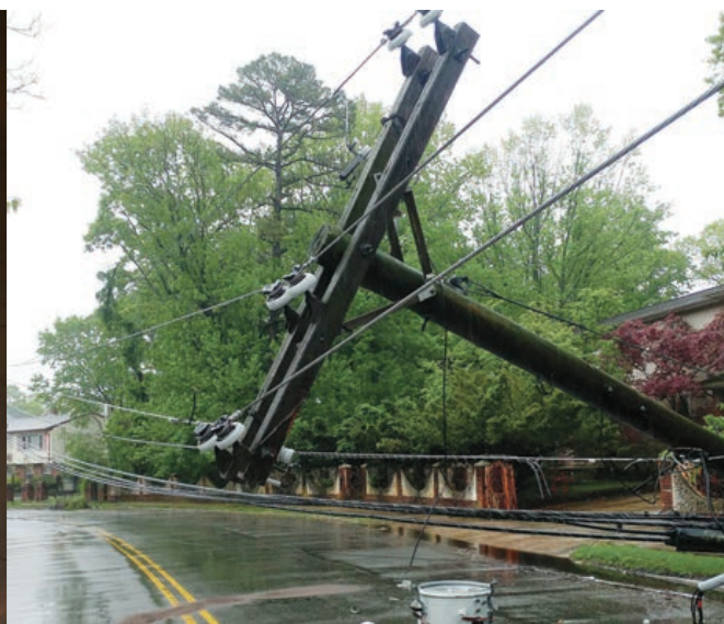
A crossarm topples, which has become more common as the number of natural disasters increases.
