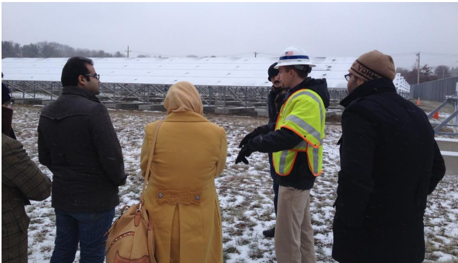
Pakistan delegation at National Grid's Haverhill 1,016kW solar generation facility. The solar PV site, situated on a former manufactured gas plant site, has 3,565 solar panels and generates enough electricity for 200 homes annually. The site serves to save approximately 1.4 million pounds of carbon from entering the environment annually.
