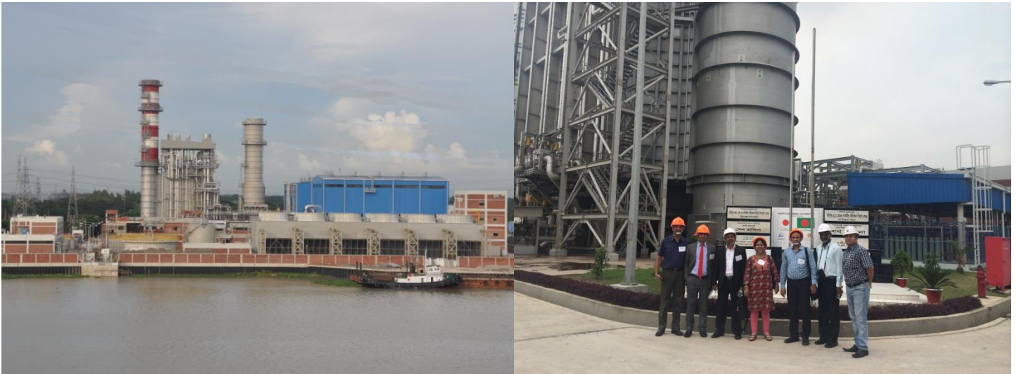
Left: The Electricity Generation Company of Bangladesh's Haripur 412 MW CCPP as seen from across the Shitalakshya River. Right: SARI/EI delegates were able to examine the difference between a simple cycle and combined cycle plant, as they toured Haripur's control room, water treatment facility, cooling towers and areas around the gas turbine, heat recovery steam generator and steam generator.
