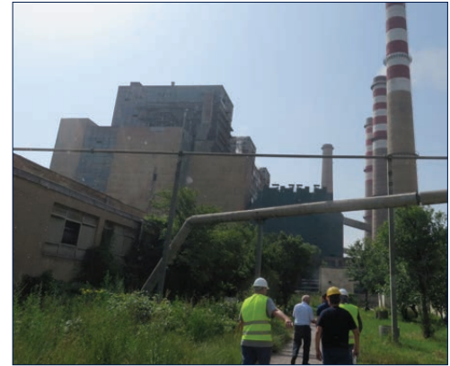
Worley Parsons team conducts Operational Assessment of Kosovo “A” power plant.
