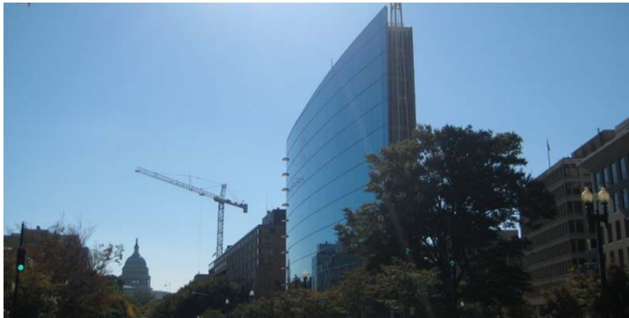
Green Building Policy
