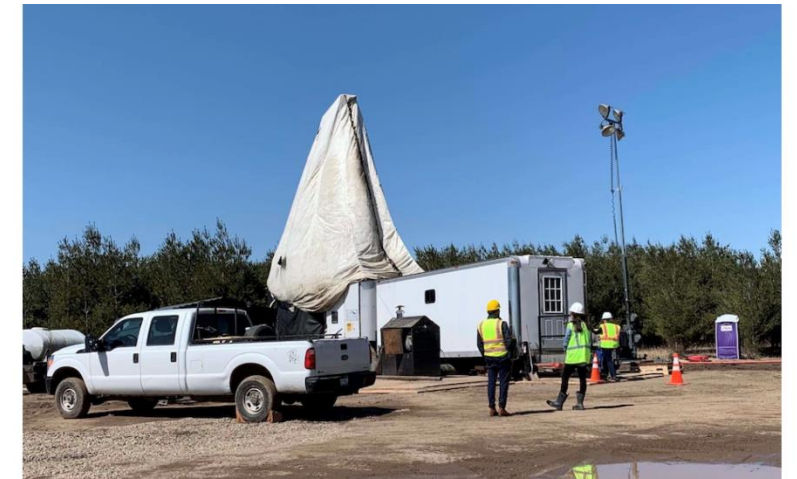
A drill rig at the Tamarack site. Photographer: Adam Minter/Bloomberg
