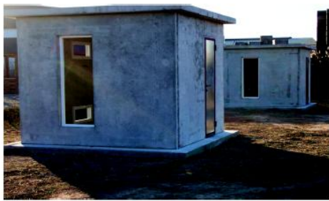
Figure 1 View of the concrete cubicles.
