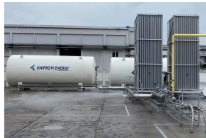
Exhibit 35. LNG storage at Uniprom-KAP in Montenegro.
