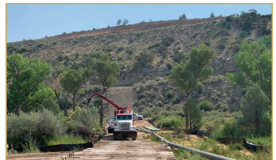
Photo: Installation of CO 2 Pipeline.
