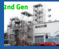
DOE/Alstom Windsor US - 3 MWth Chemical Looping, Coal
