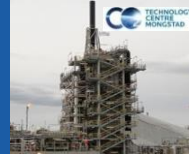
TCM Mongstad Norway 40 MWth, Chilled Ammonia, CHP RCC Offgas
