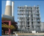
EDF Le Havre France - 5 MWth Adv. Adv. Amines - Coal
