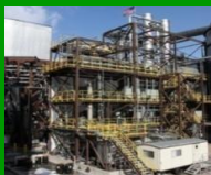
WE - Energie USA WI - 5 MWth Chilled Ammonia, Coal
