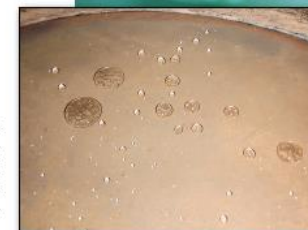
Water beads on the surface of a condenser after application of the film-forming amine
