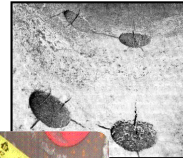
Header ID Cracking Due to Thermal Fatigue
