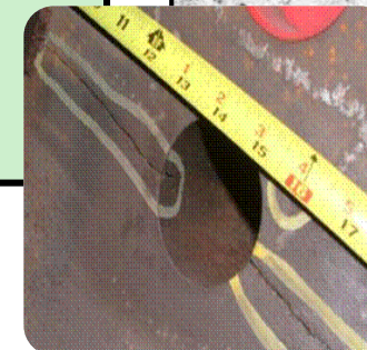
Header Fatigue Cracking
