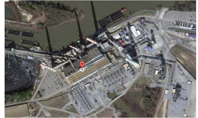
James M. Barry Electric Generating Station Alabama Power/Southern Co.
