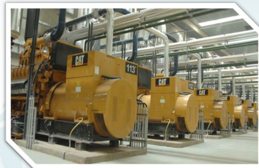
Gas power generation unit
