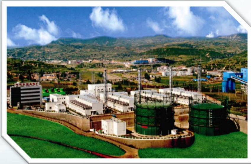
120MW gas power generation plant
