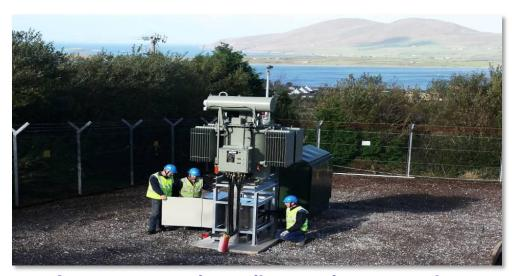
An arc suppression coil protection system has helped reduce costs; fault finding time has been reduced from 9 hours to 1.5 hours, and measured continuity of performance improved by 100%.
