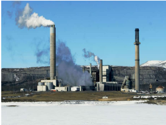
Repurposing Coal plant in Kemmerer, WY- TerraPower.
