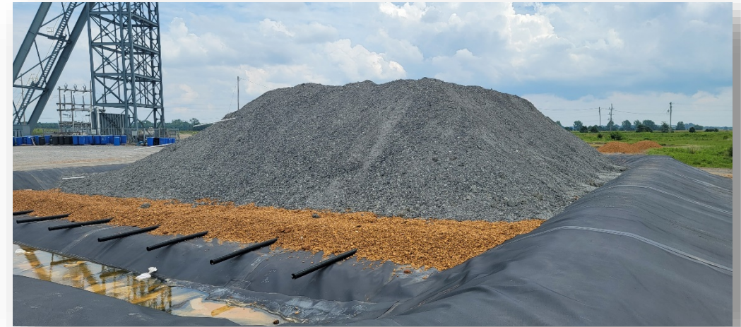
Coarse Coal Refuse Bio-Assisted Leach Pad
