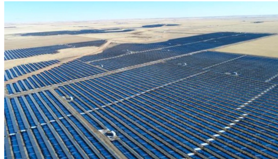
132MW Claresholm solar farm
