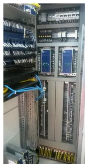
Picture 2 Inside Container
