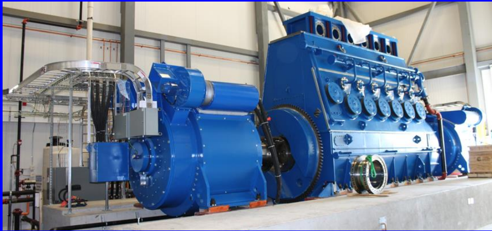
1.5MW Engine in place
