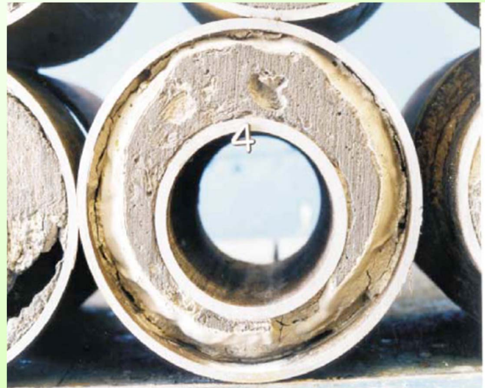
Figure 4: Incomplete displacement of drilling mud and resulting cement and drilling fluid channels. Over time, the gels in the drilling fluid well shrink, forming a gas flow path in the annulus. 3
