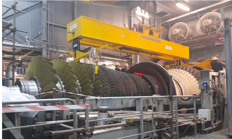
Restoration of Unit - 01
