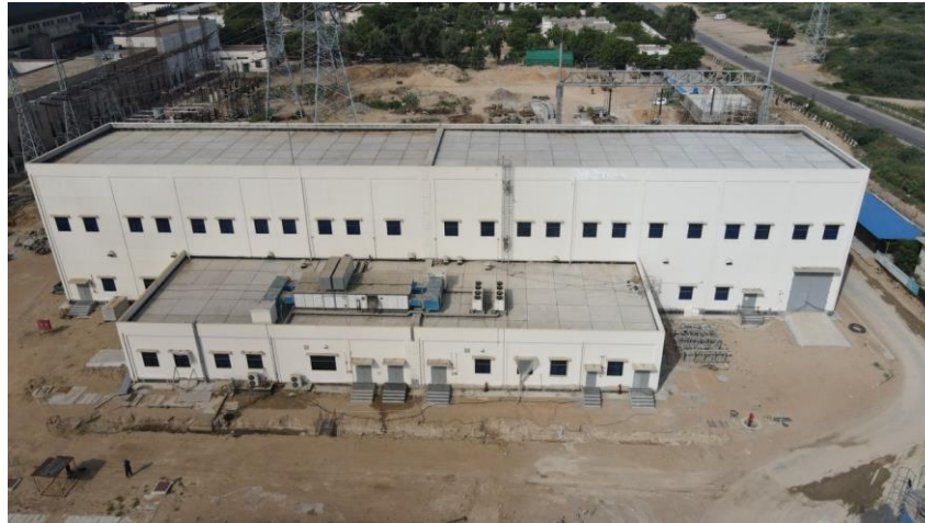
GIS and Relay Building Aerial View
