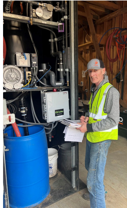
John Weyanna Treatment Plant Operator Brevig Mission
