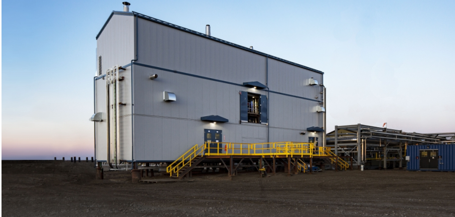
Pilot Plant Capture Unit (PPCU) at Cenovus (formerly Husky) SAGD facility in Lashburn, SK • 30 TPD • 48 Beds
