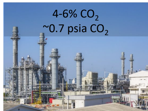
Gas Power Plant
