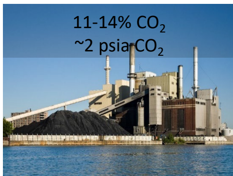
Coal Power Plant
