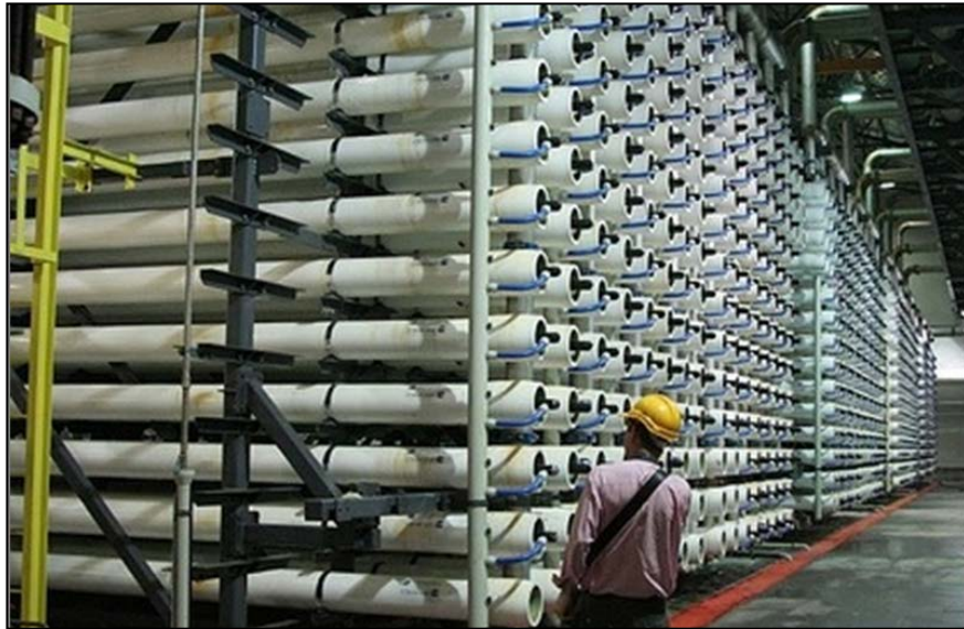
Dow Filmtec reverse osmosis system, 1.5 million m 2 area, Ashkelon, Israel
