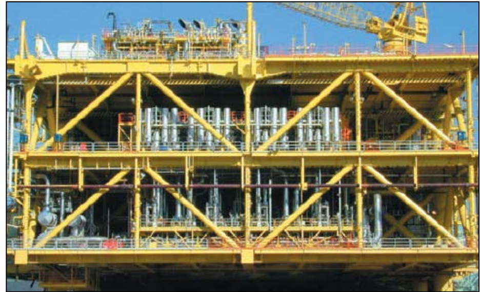
Schlumberger Cameron CO 2 /natural gas system, 700 MMscfd, Gulf of Thailand
