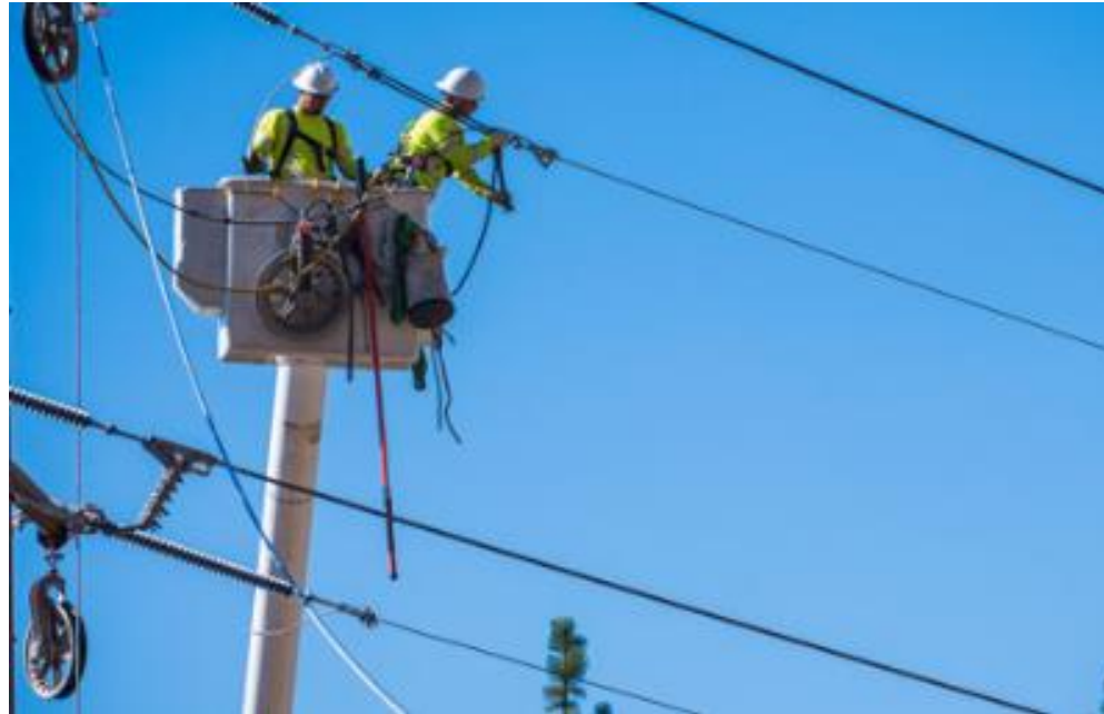
Line workers reconductoring a circuit
