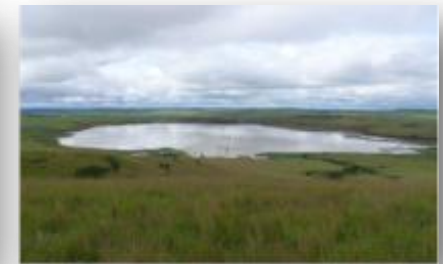
Ingula - Bramhoek dam
