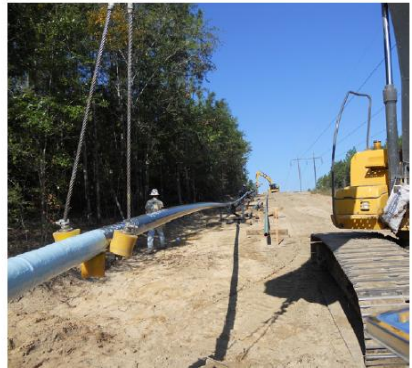
Handling pipe for horizontal directional drill
