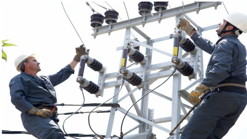
Power grid maintenance
