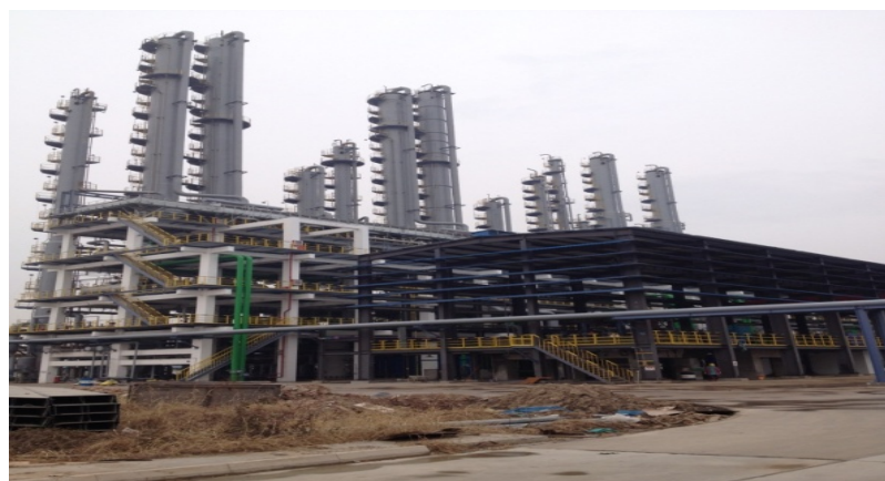
300 kt/a ethanol and iso-propanol production from acetic acid/propene as feed-stocks have done in 2015
