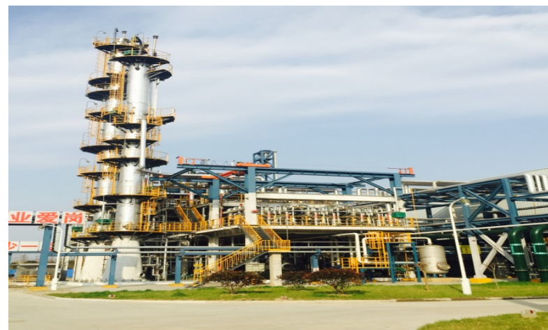
30 kt/a demon for hydrogenation of acetic acid to ethanol have done in 2016
