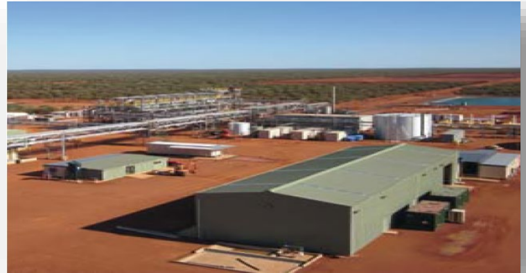
Lynas Mt. Weld REE Concentration Plant
