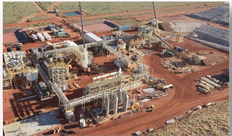
Northern Minerals Heavy REE Pilot Plant
