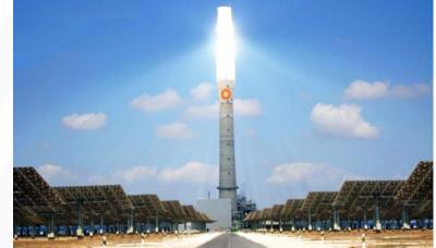
Concentrating solar power (CSP) technologies use mirrors to reflect and concentrate sunlight onto a receiver where it is collected and converted into heat. This heat energy can be stored and used to produce electricity whenever it is needed.
