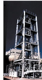
Nanko 2 metric T/D (ton per day) Natural Gas Fired CO 2 Capture Pilot Plant
