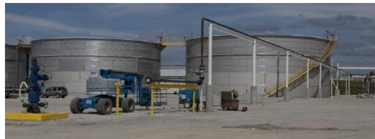
CO 2 Pipe to Injection Well
