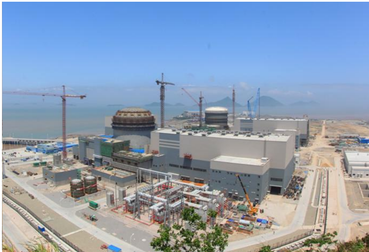
Sanmen, China AP1000 Nuclear Power Plant Construction Site
